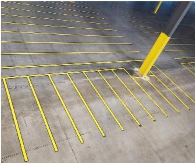
Similarly, ASG Services shot blast line striping is favored by those with a little more surety over facility layout. They can commit to a more permanent solution, so the floor is shot blasted, and a single system applied, which is a very tough option and used in some of the busiest facilities in the country. The protective clear coat can again potentially extend the lifespan to double that of the standard method.
