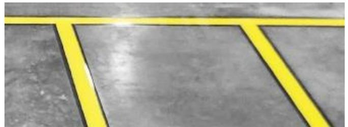
Unprepared - Direct Applied Epoxy
